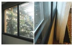
Larson's secondary window solution fit the existing windows seamlessly, reduced noise and increased energy efficiency without affecting the guests' views.
