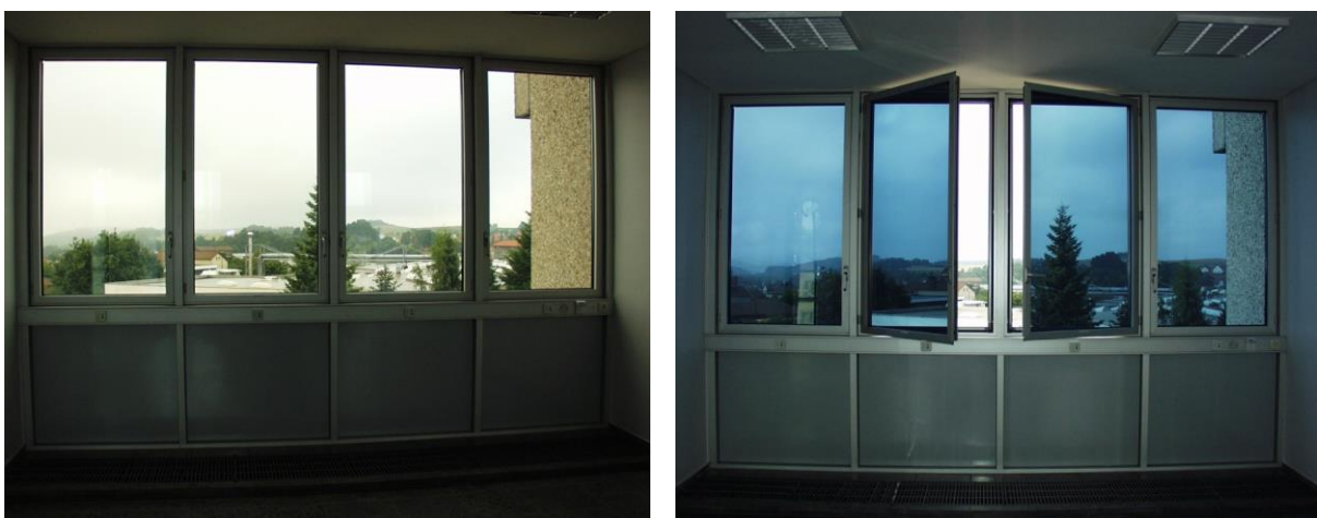
Figure 6.11 Electrochromic glazing in the clear (transparent) and darkened (blue) states.
