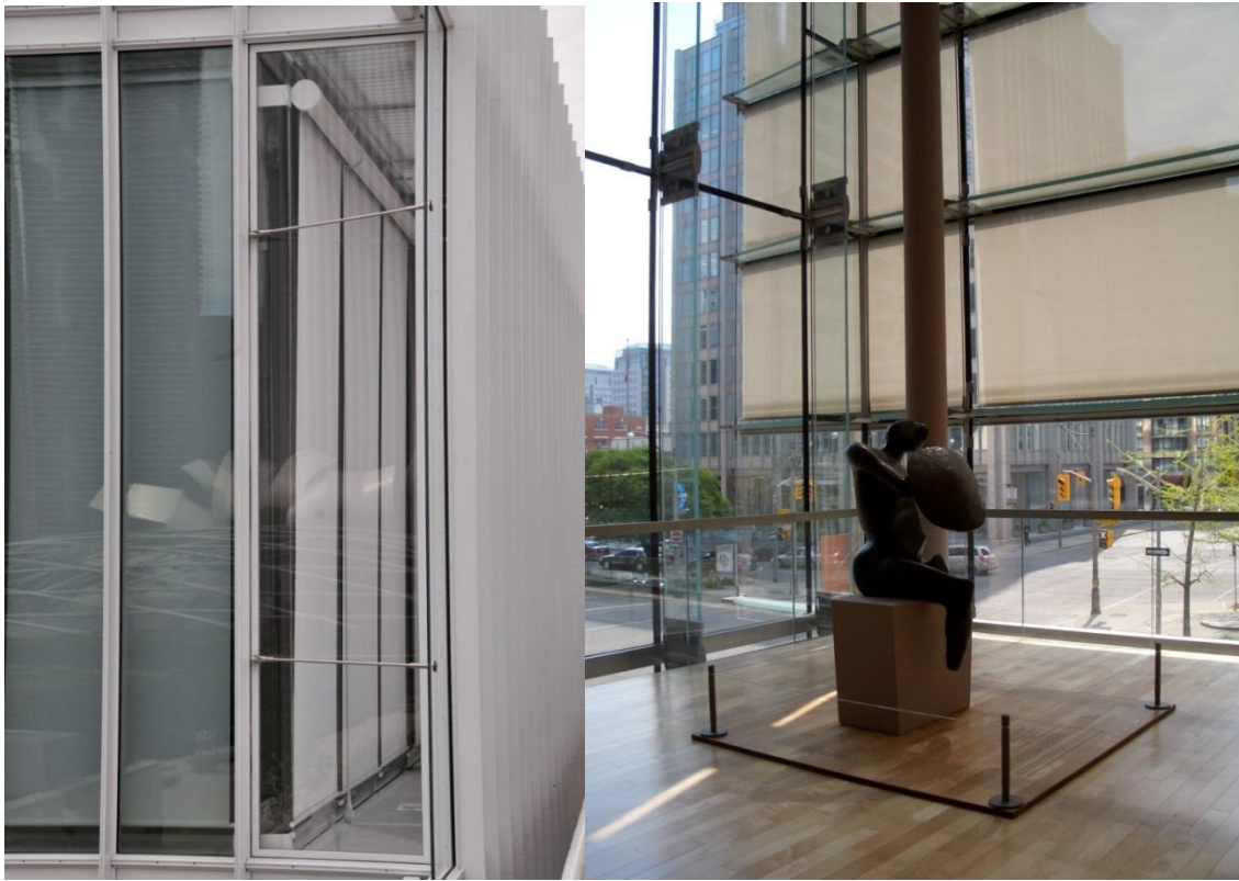
Figure 6.8 Roller shades in a double skin façade providing effective daylighting and glare control (Art Institute of Chicago, USA, photograph Wilson R (6.23)).
