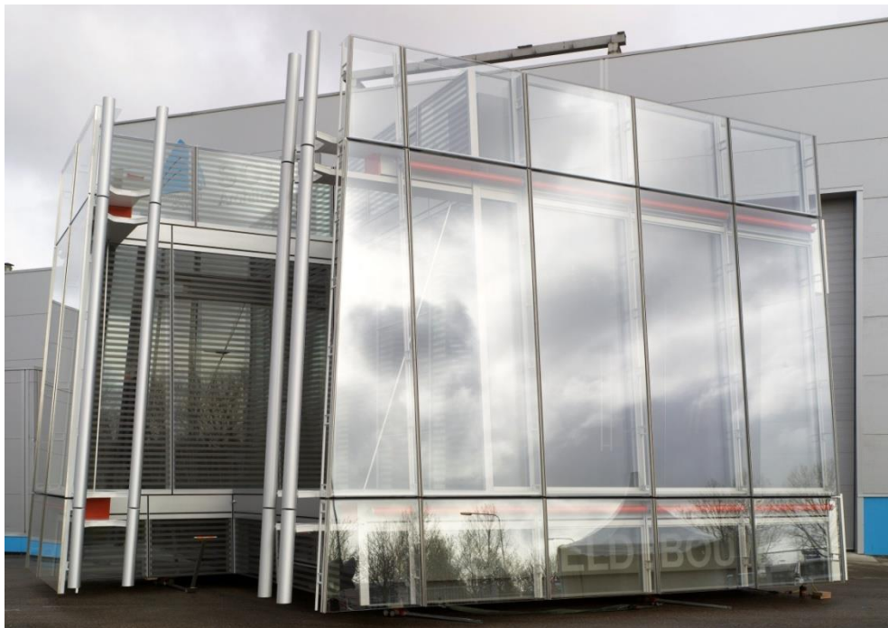
Figure 6.6 The triple-glazed system of the Shard building, London: outside single pane, ventilated inner cavity housing a motorised solar-control roller blind, inside double-glazed unit (photographs courtesy of Arup, London (6.18)).
