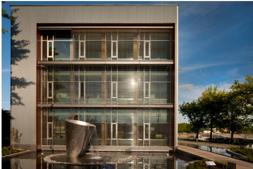
Figure 6.9 Exterior Venetian blinds (Lott Clearwater Alliance, USA, photograph Wilson R (6.23)).
