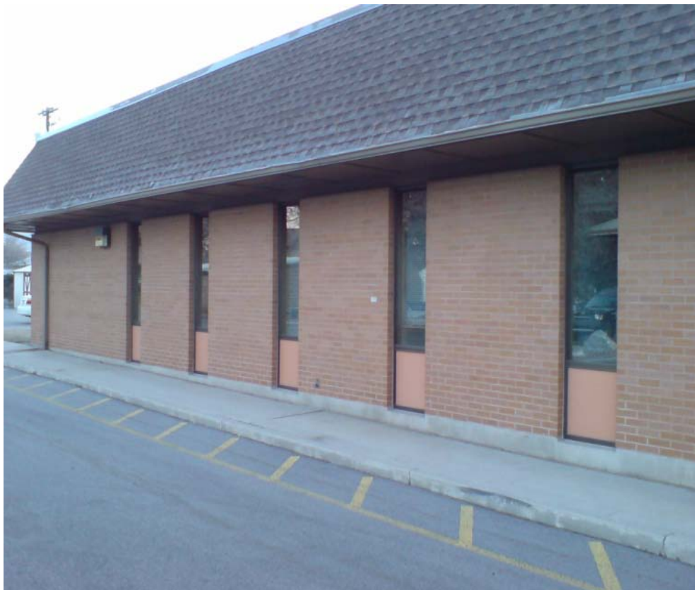
Figure 4. Exterior view of the west side of the Provo office building showing window configuration and overhang
