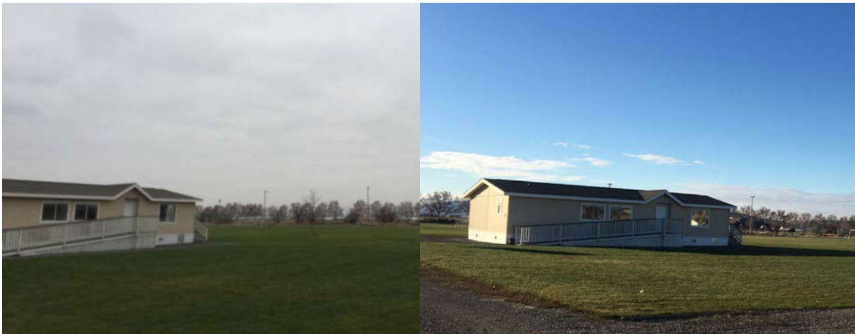
Figure 4.11. Savings Realized with Shades Pulled Down on a Cloudy Day (left photo taken on December 11, 2017, HVAC savings of 5% realized on this day). Negligible or negative average watt-hr/day savings realized on sunny days with few clouds (e.g., negative savings on December day with few clouds, right photo).
