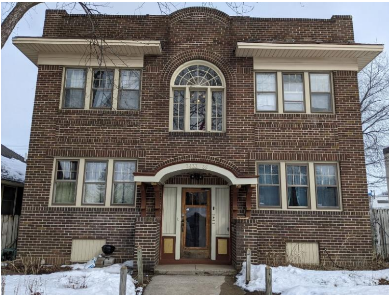
Figure 4. Site 3, “Quanta Multifamily #1,” four-plex multifamily with 55 windows, window age estimated 60–100 years. Contractor-installed product: exterior Low-E storm windows.
