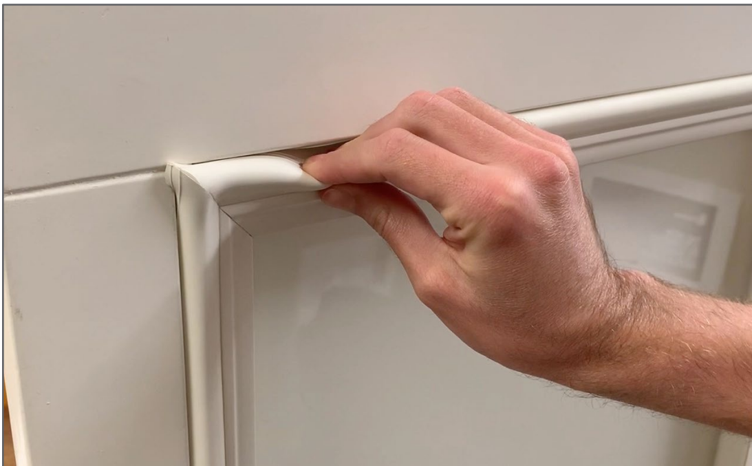
Figure: Frame-mounted acrylic panel with vinyl + weatherstripping perimeter seals
