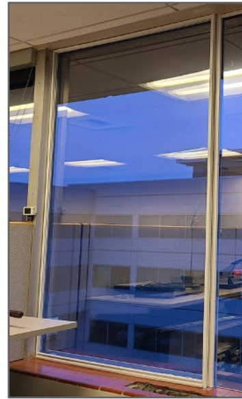
Figure: Frame-mounted acrylic panel with vinyl + magnetic perimeter seals
